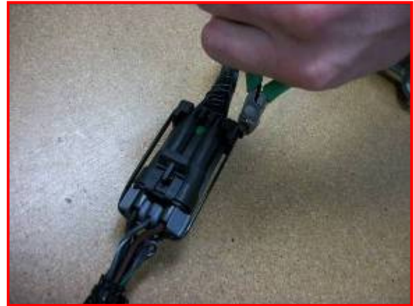
Figure 26: Zip Tie Secured and Trim
