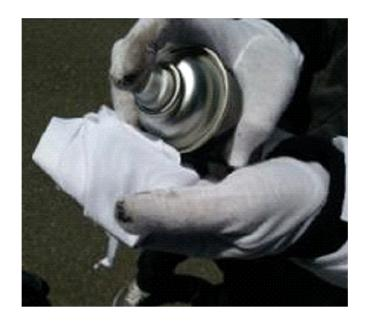
5. Wipe to remove adhesive residue using 3M Premium Sticker Cleaner – MS061 or equivalent if available.
