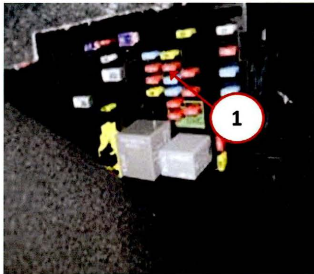
Fig. 4 JC Passenger Side Fuse Block
