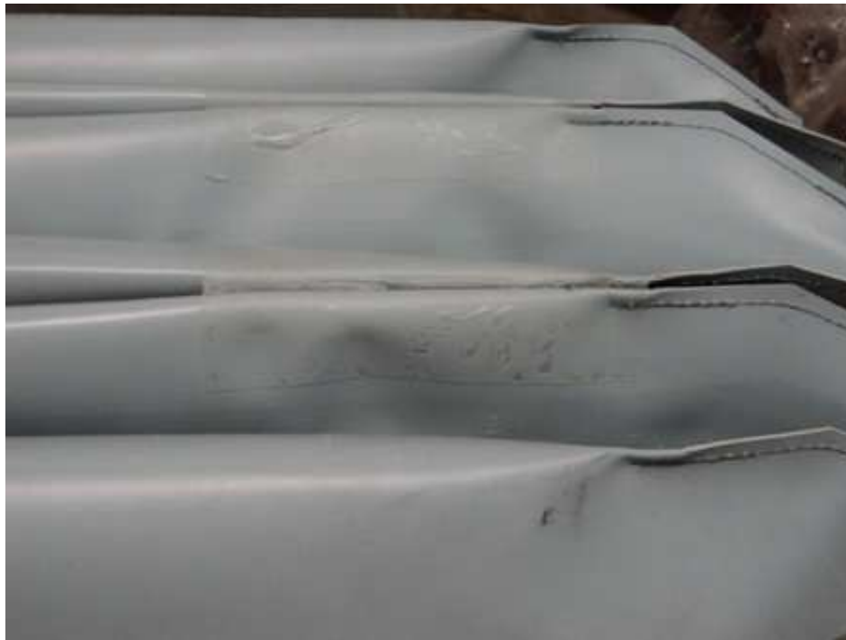
Figure 3: FALSE CEILING BELLOWS REPAIR (TAPE INSTALLED ON TWO FOLDING SECTION)
