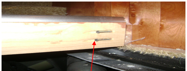
Fig. 2—Remove lower wardrobe track.
