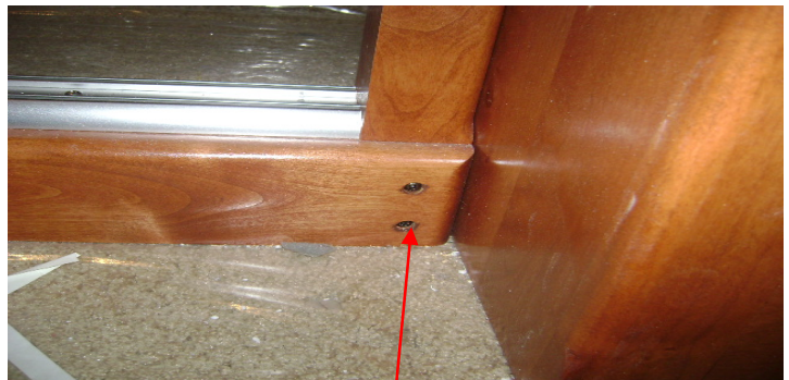
Fig. 1—Remove screws from the toe kick.
