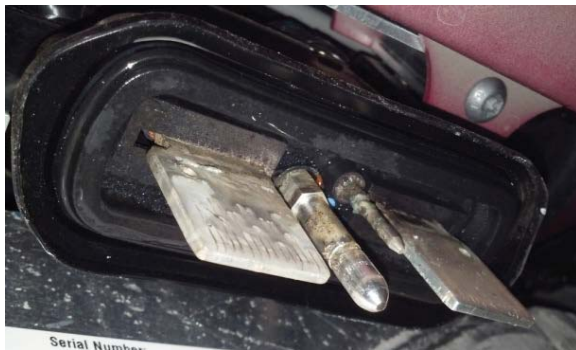
Figure 22 (Arcing and corrosion on vehicle side Rapid Mate)
