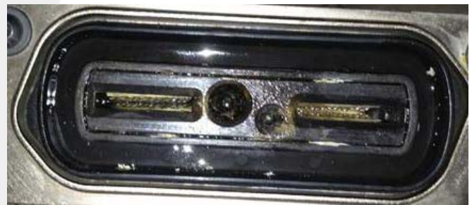
Figure 23 (Significant amount of water in battery side Rapid Mate)
