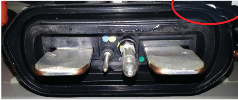
Figure 19: Example of Compromised Outer Skirt
