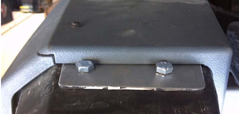
Cladding snug against lower bolts (viewed from below)
