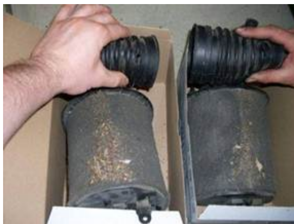
Figure 1. Example of excessive dirt on air filters.
