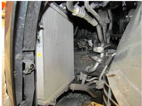
Figure 9. Charge air cooler exit air duct installed.
