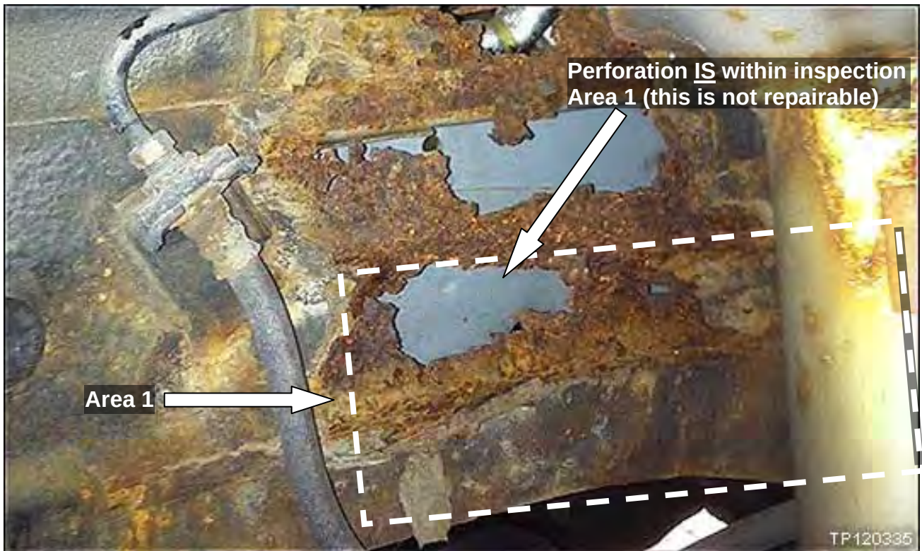
Example (Additional Photo) of Area 1 Perforation Inspection
