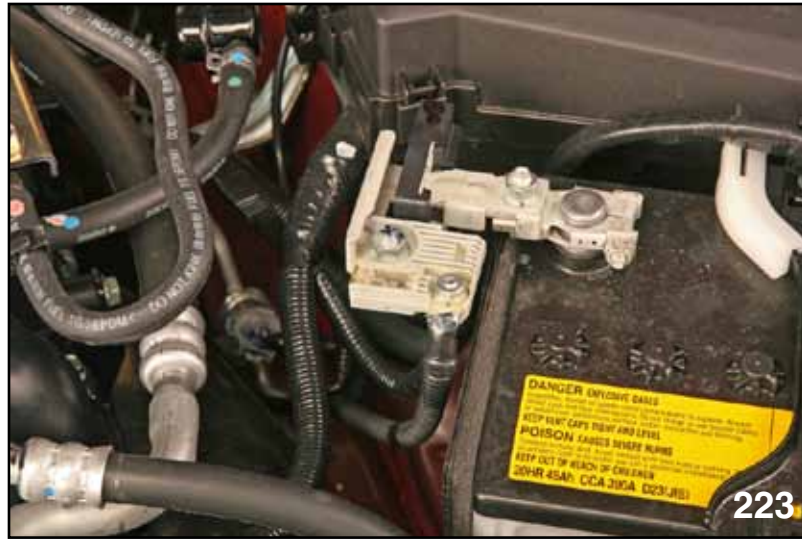
AMP Clamp Positive Battery Post
