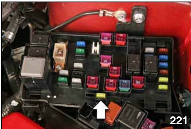
Back Up Power Supply Fuses
