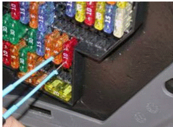
Figure 1. Measuring voltage drop across a fuse.
