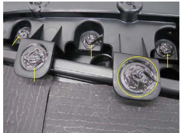
Figure 5. Weld points of the door panel.
