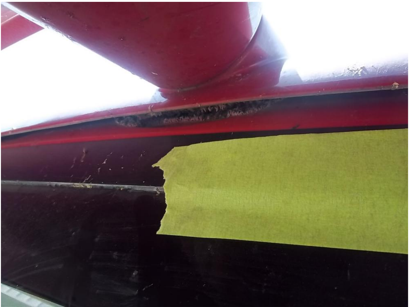
The sunshade mounting bracket is starting to come loose from the vehicle - the adhesive patch at the center mount is pulling apart.
