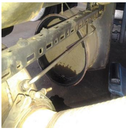
DPF Outlet Coolant - Oil Contaminated
