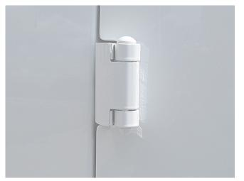
The door hinges and pins may be binding or seized, due to internal corrosion. This condition is most commonly noted with the original hinge design shown above.
