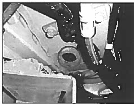
Figure 4. Rear Tie-Down Location - After Installation
