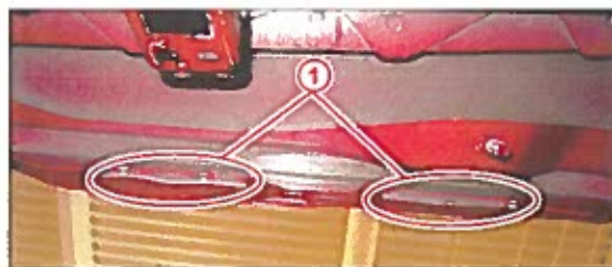
1 Example of Installed Shims
