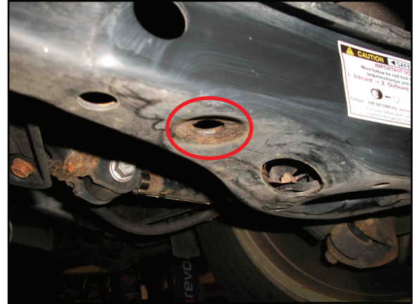
Figure 2. Stabilizer Link Damaged
