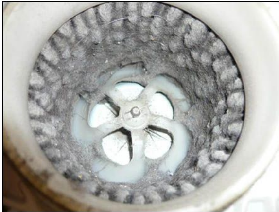
Figure 1. HV Battery Cooling Fan BEFORE Cleaning
