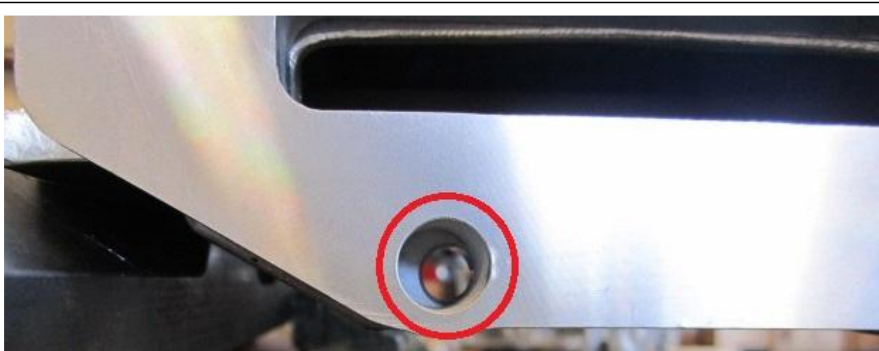
Red circle is the area of concern
