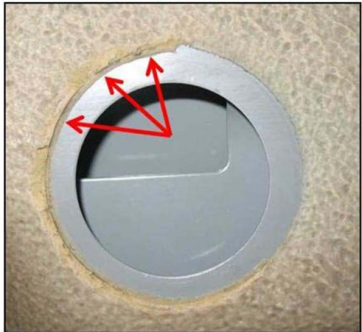
Figure 2. Red arrows indicate excess underseal.
