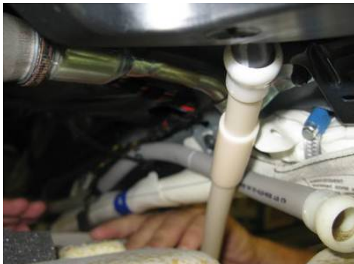
Figure 1. Disconnect original drain.
