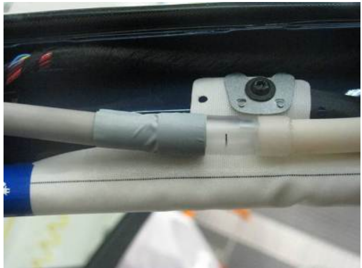
Figure 15. Wrap tape around connection.
