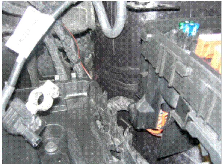
Figure 3. Routing up from Central Electrics.
