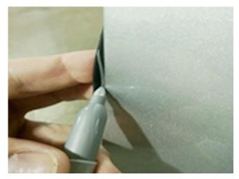
3. Following the edge of the door, use a white pen or marker to trace a line onto the outside of the weatherstrip.
