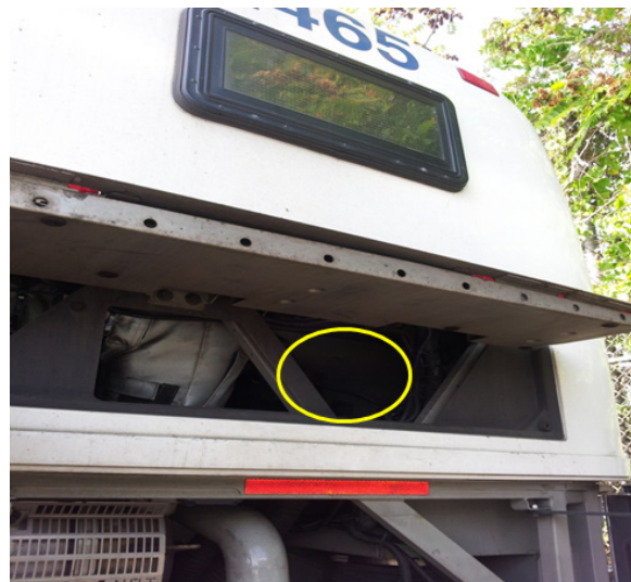
NEW HARNESS WILL END UP HERE AT S-BAR 1 SPLICE BAR CONNECTOR
