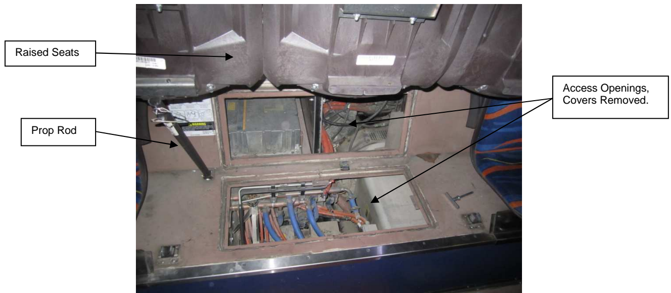
Figure 1: Access Openings Under Chesterfield Seats.
