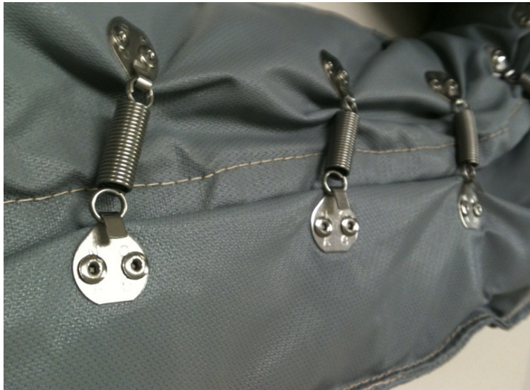
Figure 2: Insulated Blanket Installation
