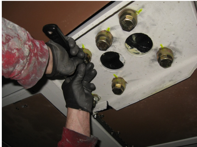
Figure 7: Scrape Away Old Torque Marks
