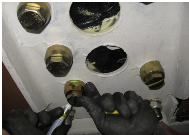
Figure 9: Re-apply Torque Marks
