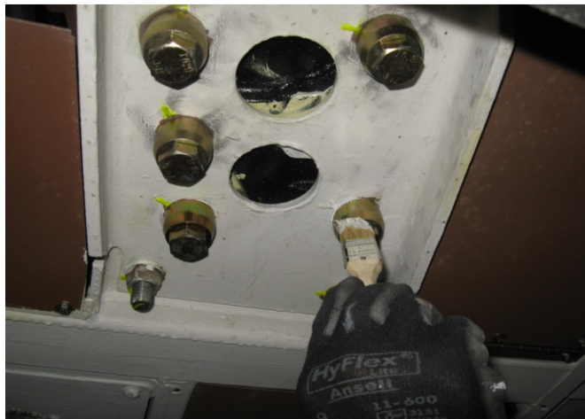
Figure 8: Touch up Primer and Corashield
