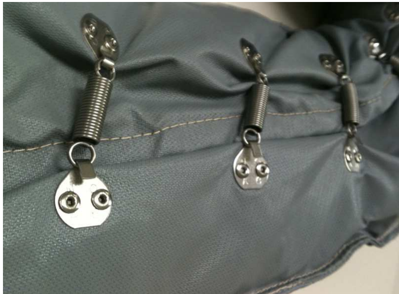
Figure 4: Insulated Blanket Installation
