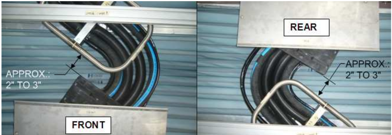
Figure 8: BLACK PLASTIC WEAR PLATE INSTALLATION
