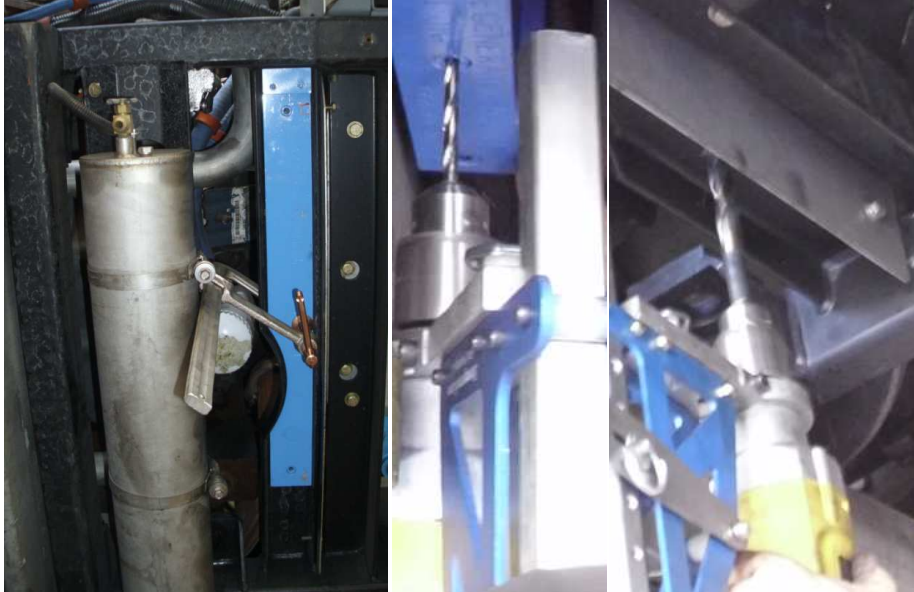
Figure 18: CS Mount Drilling
