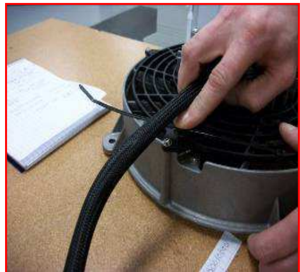
Figure 14: Installing Zip Tie into Guard
