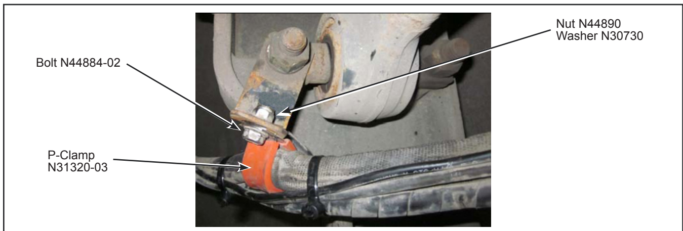
Figure 8 - L Support and P-Clamp Installation
