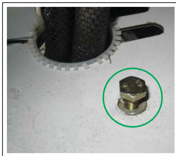
Figure 2 - Emergency Door Release Cable Box Bolt
