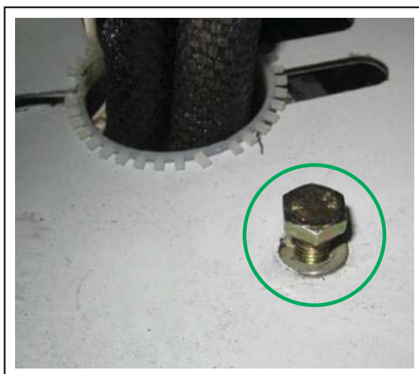
Figure 2 - Emergency Door Release Cable Box Bolt
