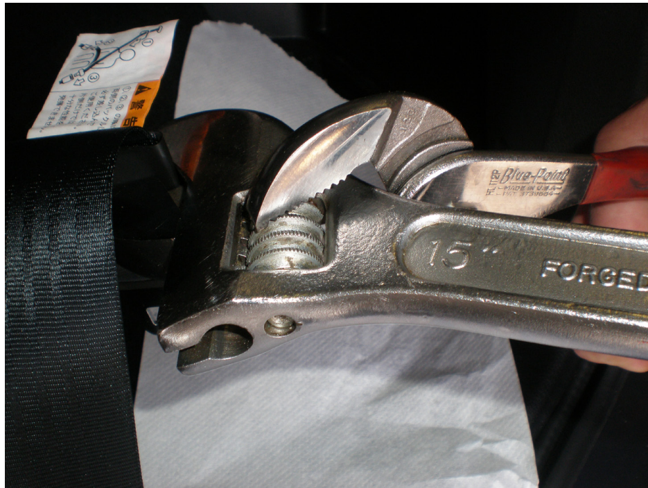
Figure 9: Seating the Tack Collar
