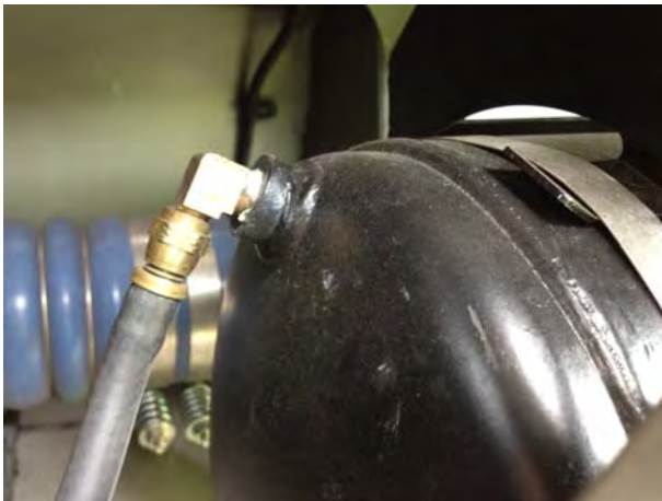
NEW COOLANT SURGE COOLANT SURGE TANK INSTALLED - ROAD SIDE
