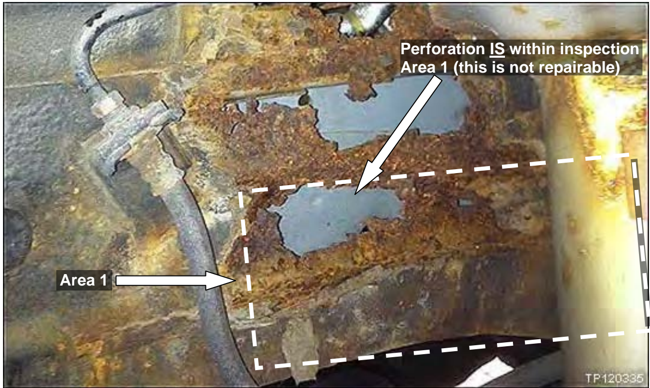
Example (Additional Photo) of Area 1 Perforation Inspection
