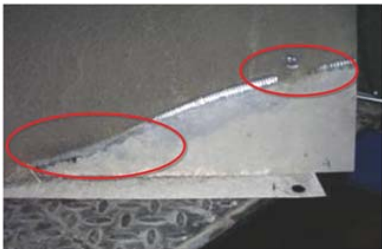
Figure 2 Evidence of Contact (Cable/Harness/Hose) with Air Management Panel
