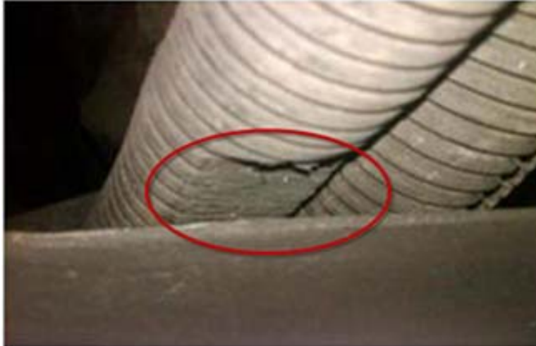
Figure 1 Battery Cable or Harness Conduit Abrasion
