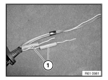
37. Slide a shrink tube (1) over each wire.
