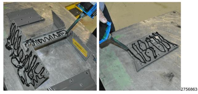
**Caution:** Ensure the Pliogrip two-part polyurethane mix is uniform in color BEFORE applying it to the parts. Discard the first 25 mm (1 in) of the mix that is not uniform. The color of the polyurethane varies. The illustrations in this bulletin show the polyurethane mix in black or green. The Pliogrip two-part polyurethane has a 30-minute open time. The application of the Pliogrip two-part polyurethane and the assembly of the reinforcement assembly must be completed in 30 minutes.
