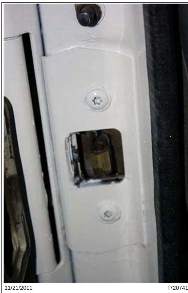
Fig. 7, Door Jamb Patch Plate Installed
