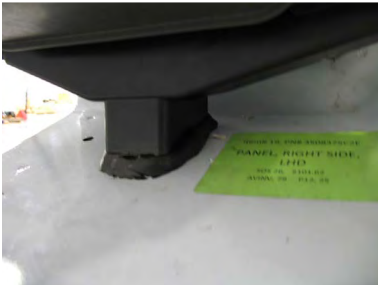
Figure 30 Sealing HVAC unit to the Floor
