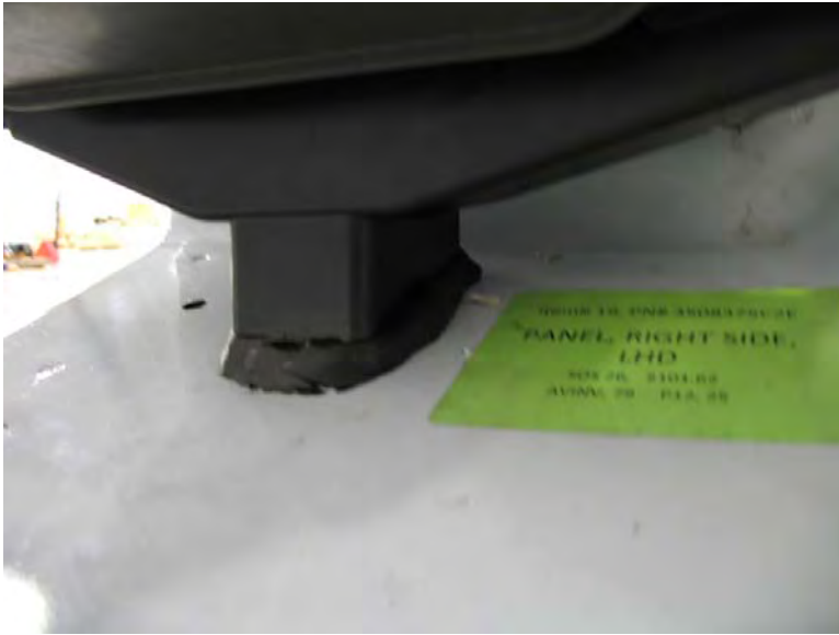
Figure 25 Sealing HVAC Unit to the Floor
