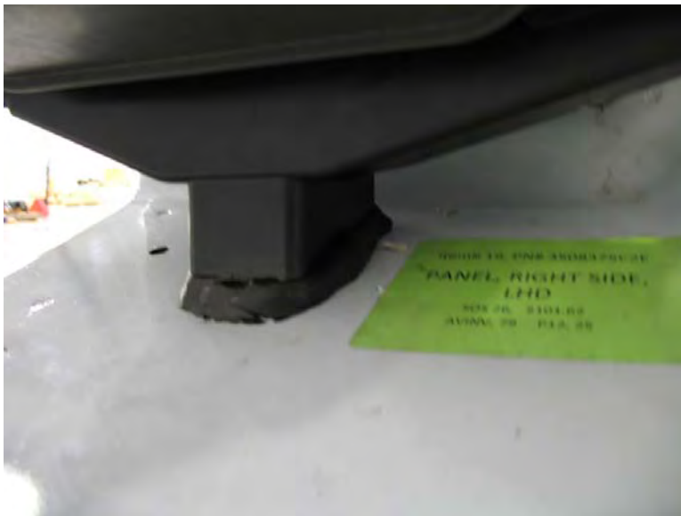
Figure 9 Sealing HVAC Unit to the Floor
