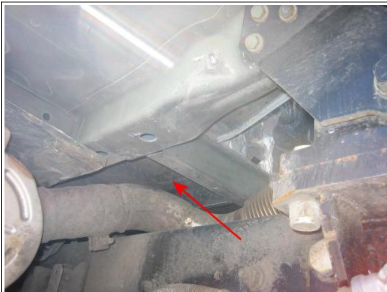
Photo 1 - Cab Floor Insulator Location - Right side
