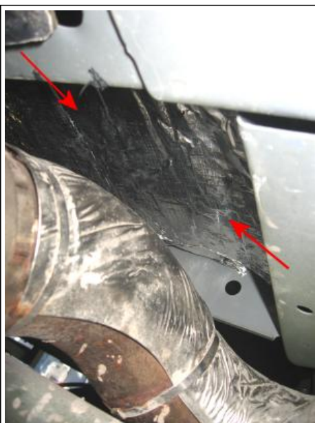
Image 5 - Heat Shield Installed
