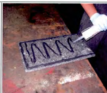
Image 4 - Properly Apply Adhesive
