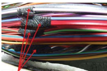
Photo 6: Add extra electrical tape at the damage points
