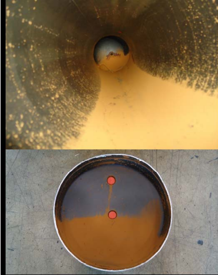
Figure 2 – Vehicle Air Tanks With Rust
